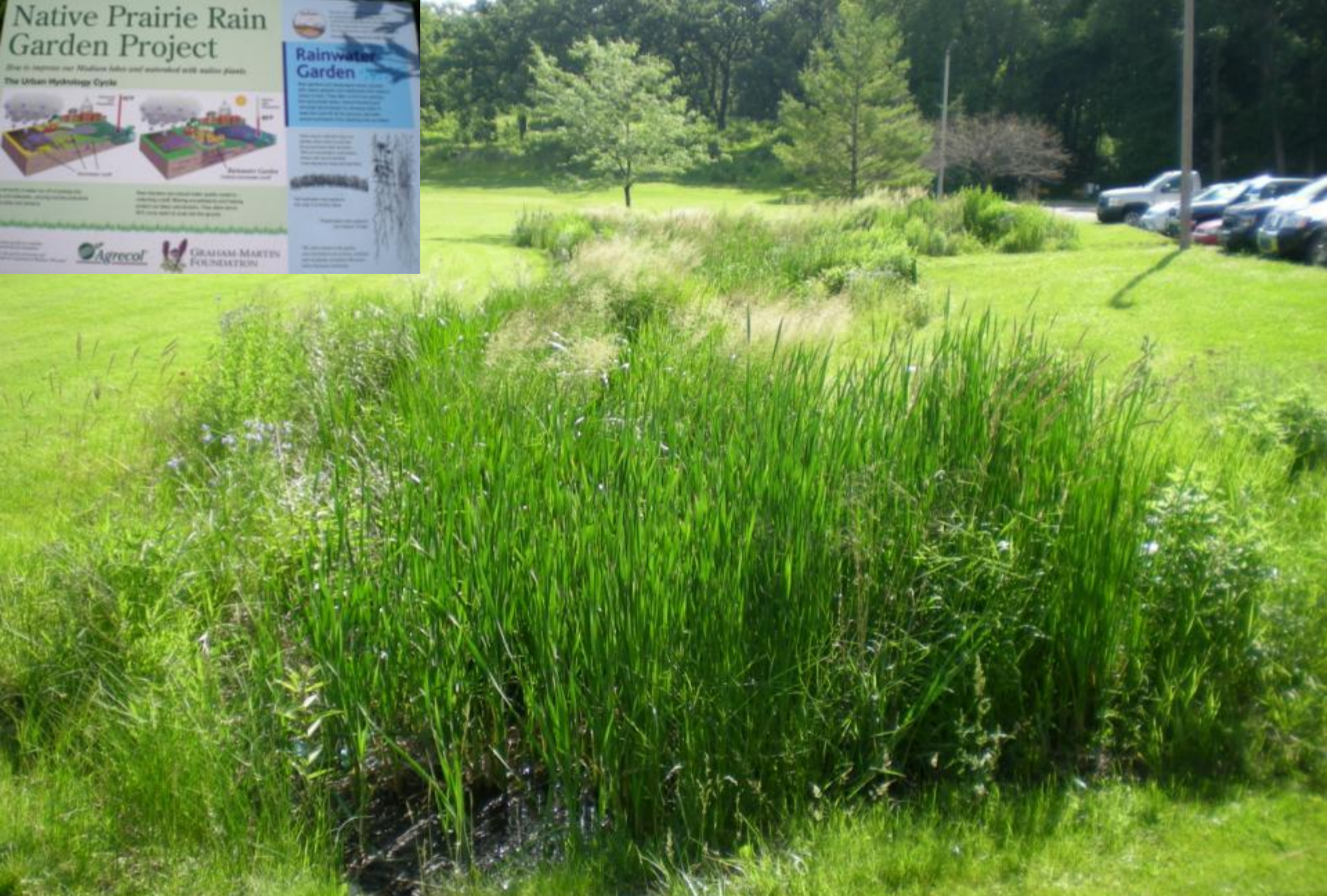
Treatment of stormwater runoff in a „Water Garden“, Madison, Wisconsin
